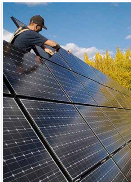
Photo: Installing solar panels (Gordon Howell).
