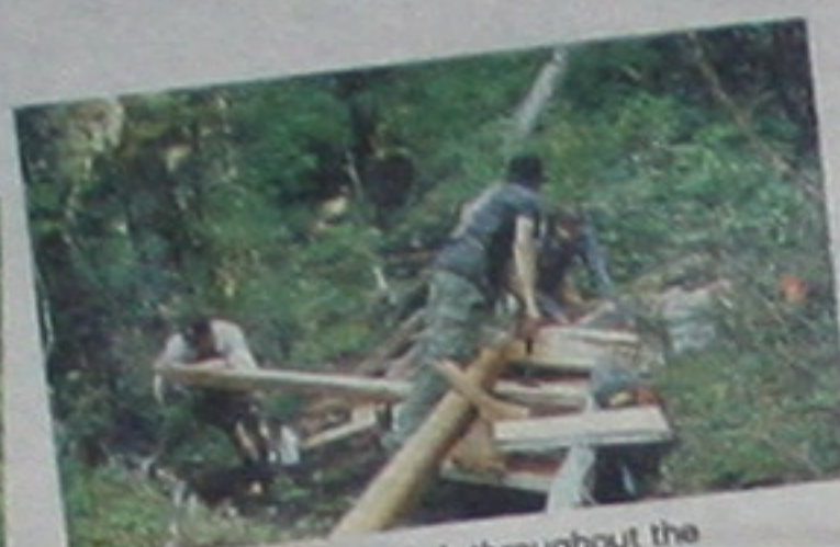
WCWC volunteers work throughout the summer of 1993 to construct the Clayoquot Valley Witness Trail. Boardwalk is constructed in order to protect the delicate forest soils from impact by hiker's boots. The trail is built under the guidance of the Tla-o-qui-aht First Nations. Photo by Joe Foy.
