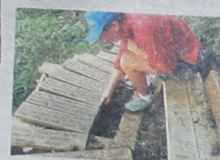
WCWC volunteers work throughout the summer of 1993 to construct the Clayoquot Valley Witness Trail. Boardwalk is constructed in order to protect the delicate forest soils from impact by hiker's boots. The trail is built under the guidance of the Tla-o-qui-aht First Nations. Photo by Joe Foy.
