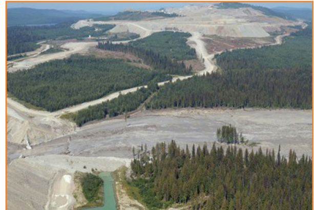
Mount Polley tailings dam failure.
