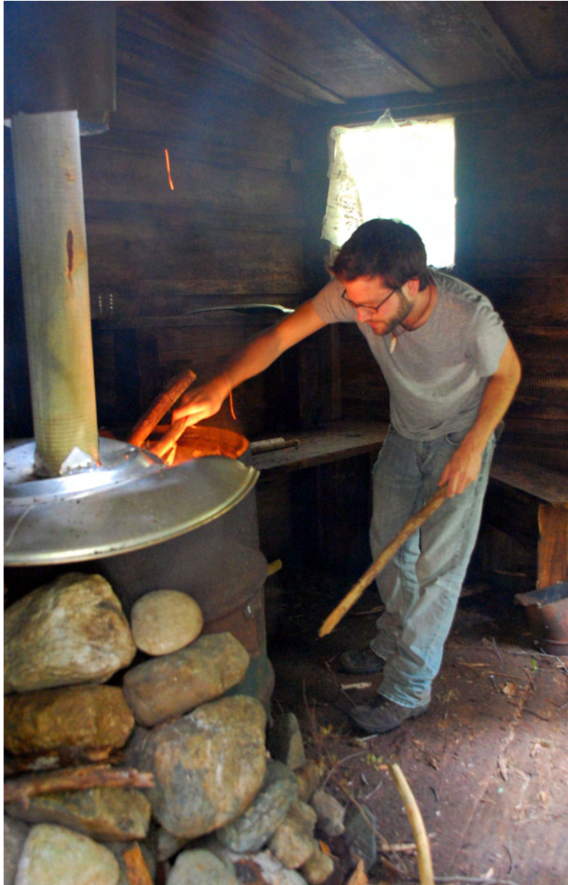
Inside of sauna. Rusted drum stove and stove pipe need replacing, as well as some rotten floor boards and central posts and beams.
