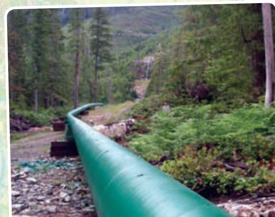
River-diversion pipe at Marion Creek Power Project (between Port Alberni and Tofino).
