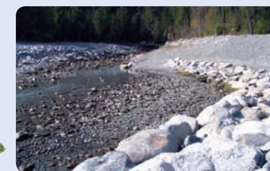
...and Miller Creek during the critical low-water incident (September 8, 2007).
