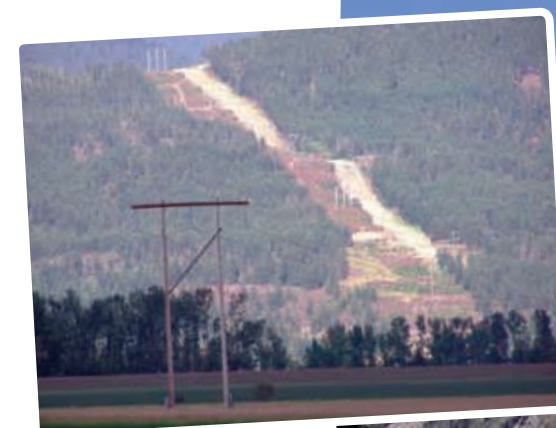
Transmission lines accompany the development of all private hydro projects. Photo: Gary Diers.
