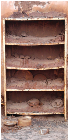
INTERIOR OF BUILDING IN BENTO RODRIGUES, THE TOWN CLOSEST TO THE MARIANA TAILINGS DAM. NOVEMBER 2016, ONE YEAR AFTER THE BREACH. PHOTO: MIGUEL FERNANDES FELIPPE, TERRA / UFJF.
