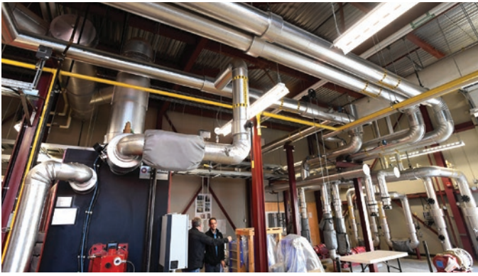
The City of Prince George Downtown Renewable Energy System (Prince George Citizen Staff)
