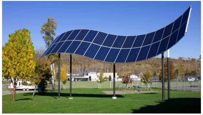
Hudson Hope community solar initiative installed solar panels (Peter McCartney)
