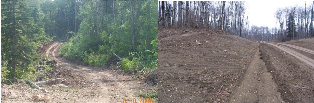
Figure 8.22 Forest road narrow right of way (left) unstumped; (right) stumped.
