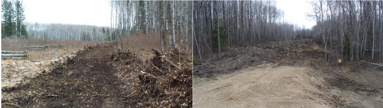
Figure 8.9 Roadside pile of organic soil, roots, and stumps (left). Organic soil spread back over a decommissioned road (right).
