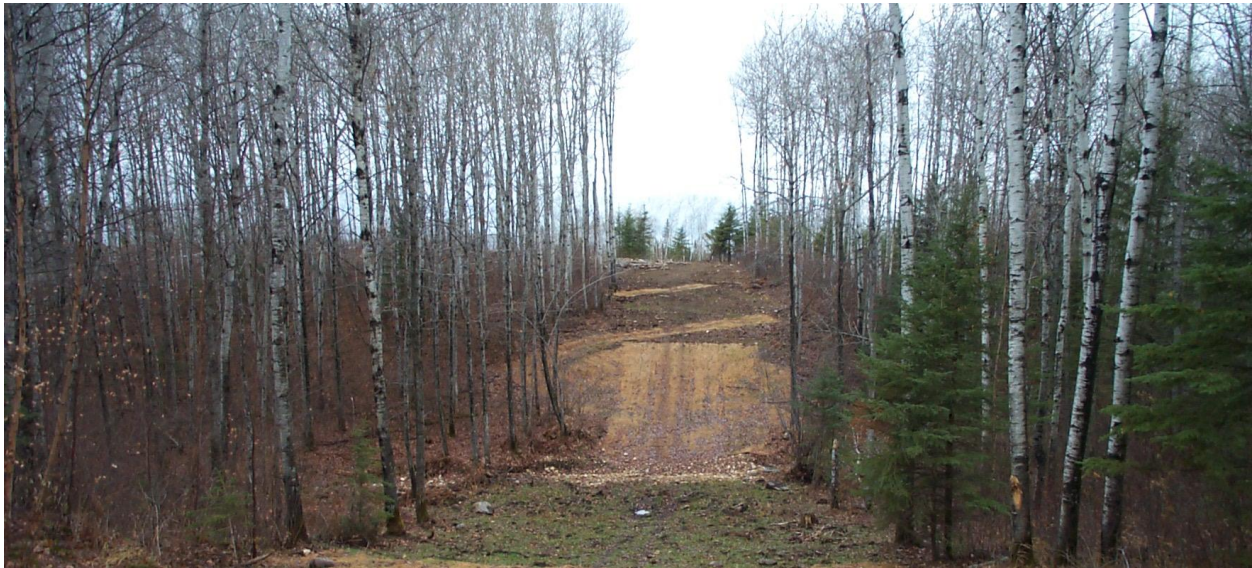
Figure 8.25 Decommissioned crossing with erosion control.
