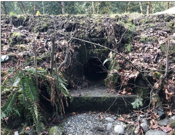
Photo 5. Culvert outlet leading to the Goldstream River, upstream view.
