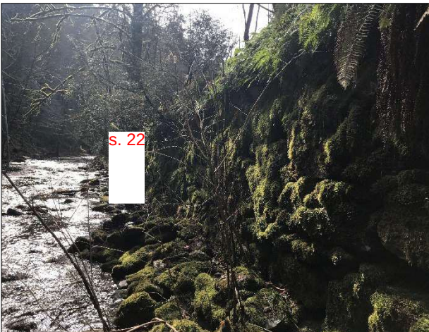
Photo 6. Example of the stone stacked wall, south view
