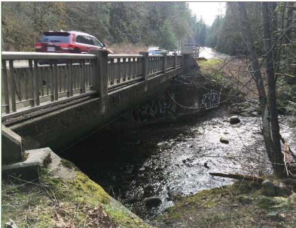
Photo 3. Goldstream River Bridge, south end of the alignment, north view.
