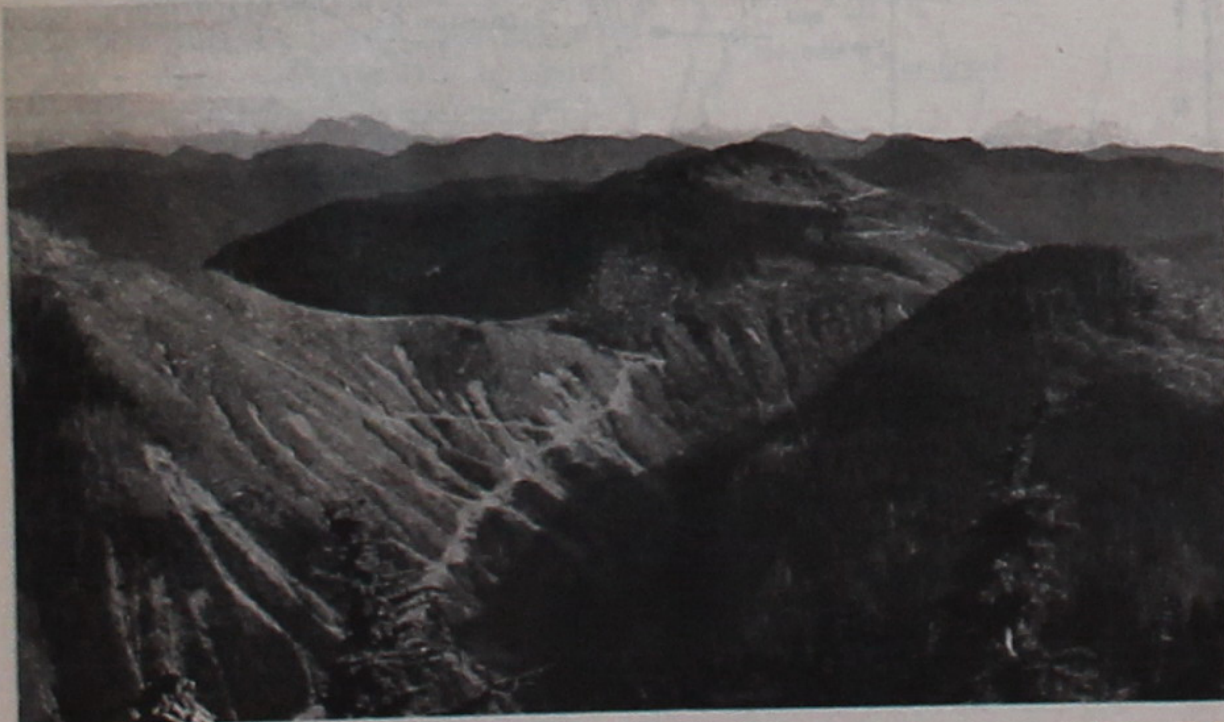
Cascade Creek, northeast of Mission B.C. Entire valley and ridge tops clear cut. Note all the mudslides caused by logging. The resulting flash flooding in the lower part of the creek caused a great deal of damage to homes and property. Photo: Ken Lay
