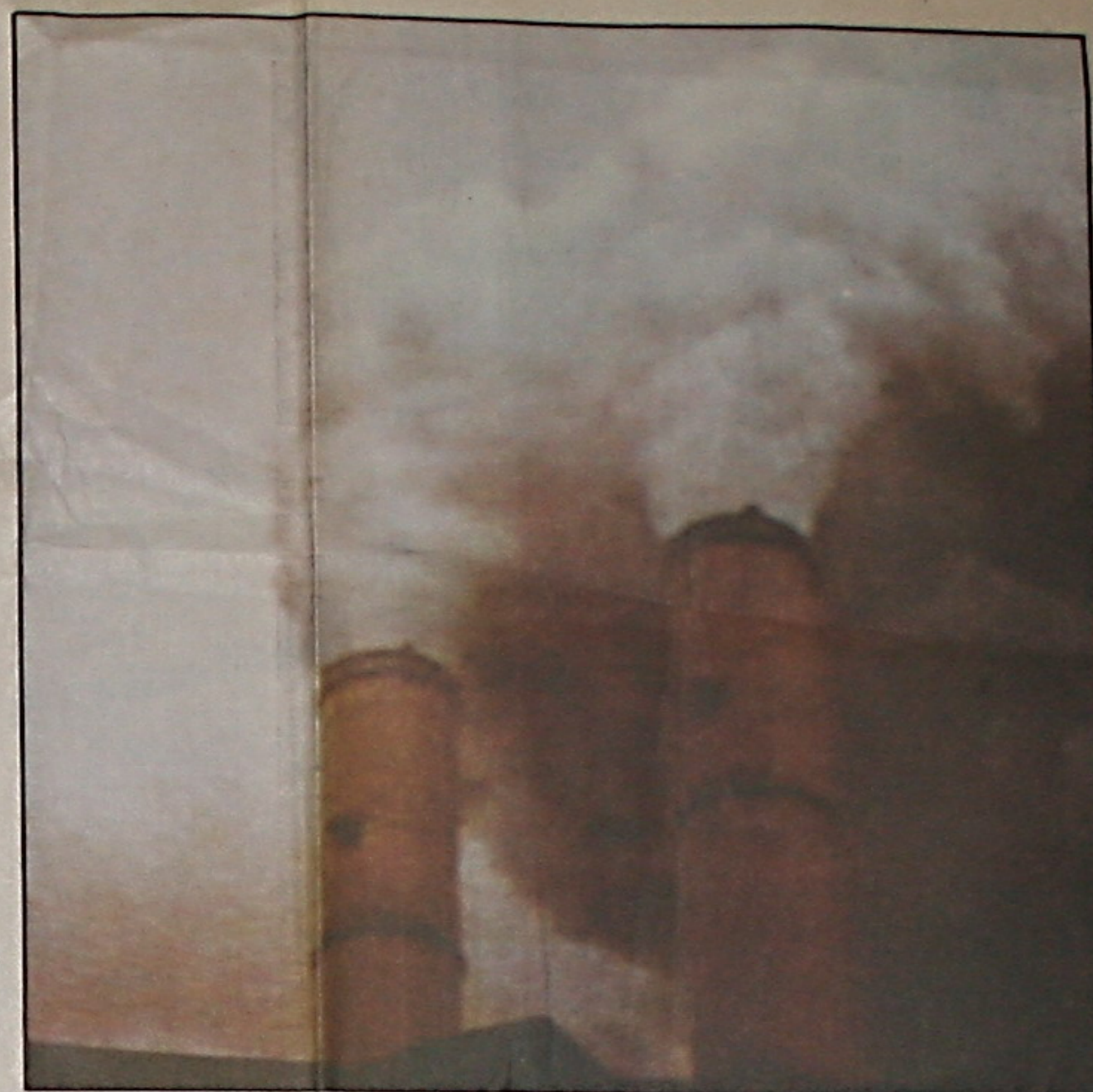
above - This 1989 photo shows the emissions from two of the three recovery boilers at Canfor's Port Mellon mill. According to Environment Canada, the pulp and paper industry is the most toxic industry in Canada, producing more than 1,000 toxic compounds. Some of them have yet to be identified. The U.S. Environmental Protection Agency claims that particulate ash from pulp mills is a carrier of sulphur dioxide and dioxins. Dioxins, clinging to dust and smoke particles, can be absorbed through the lungs directly into the bloodstream. Sulphur dioxide converts into sulphuric acid when inhaled into the lungs.
