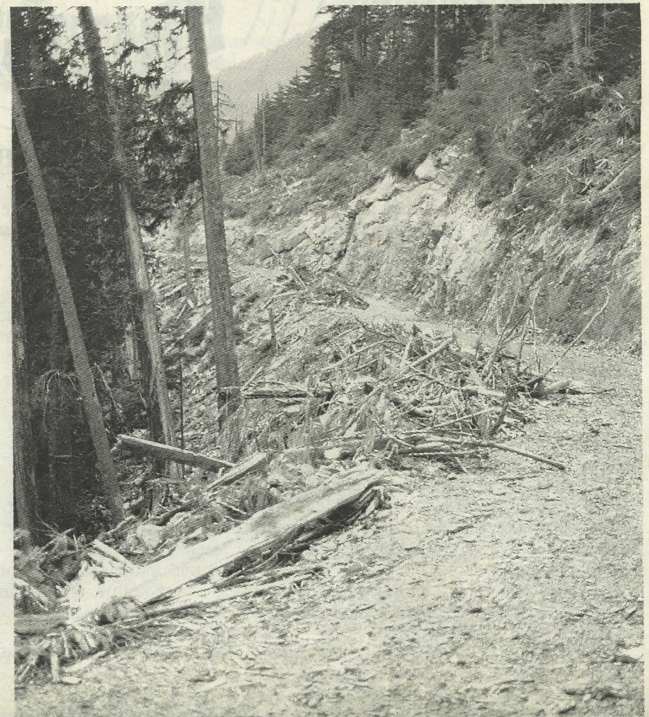
Newly built road into Boise Valley in preparation for clearcut logging
