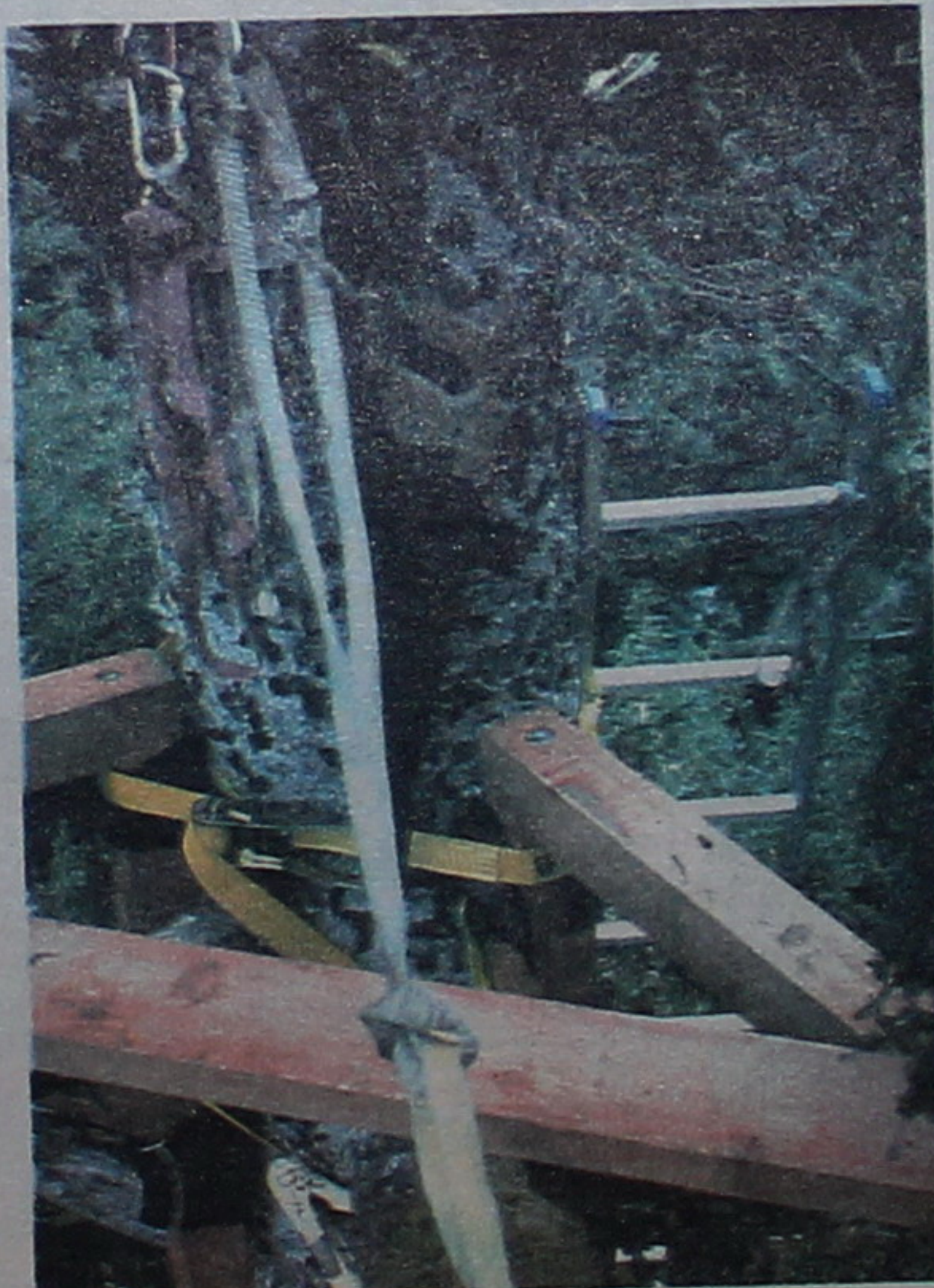
Construction detail of removable braces
