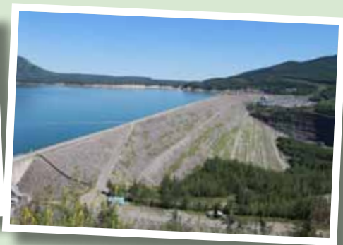
Photo: WAC Bennett dam (Joe Foy).
